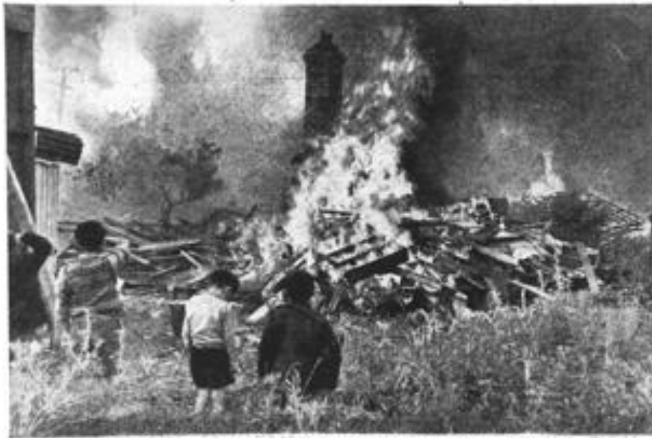
One of the ramshackle homes at Orakau set on fire after demolition yesterday.
