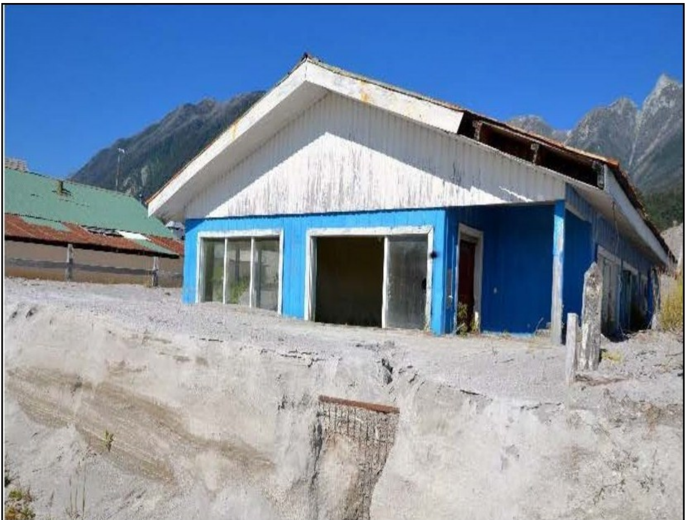
An abandoned house in the centre of Chaitén township partially buried by ash from the 2008 eruption of Chaitén Volcano
