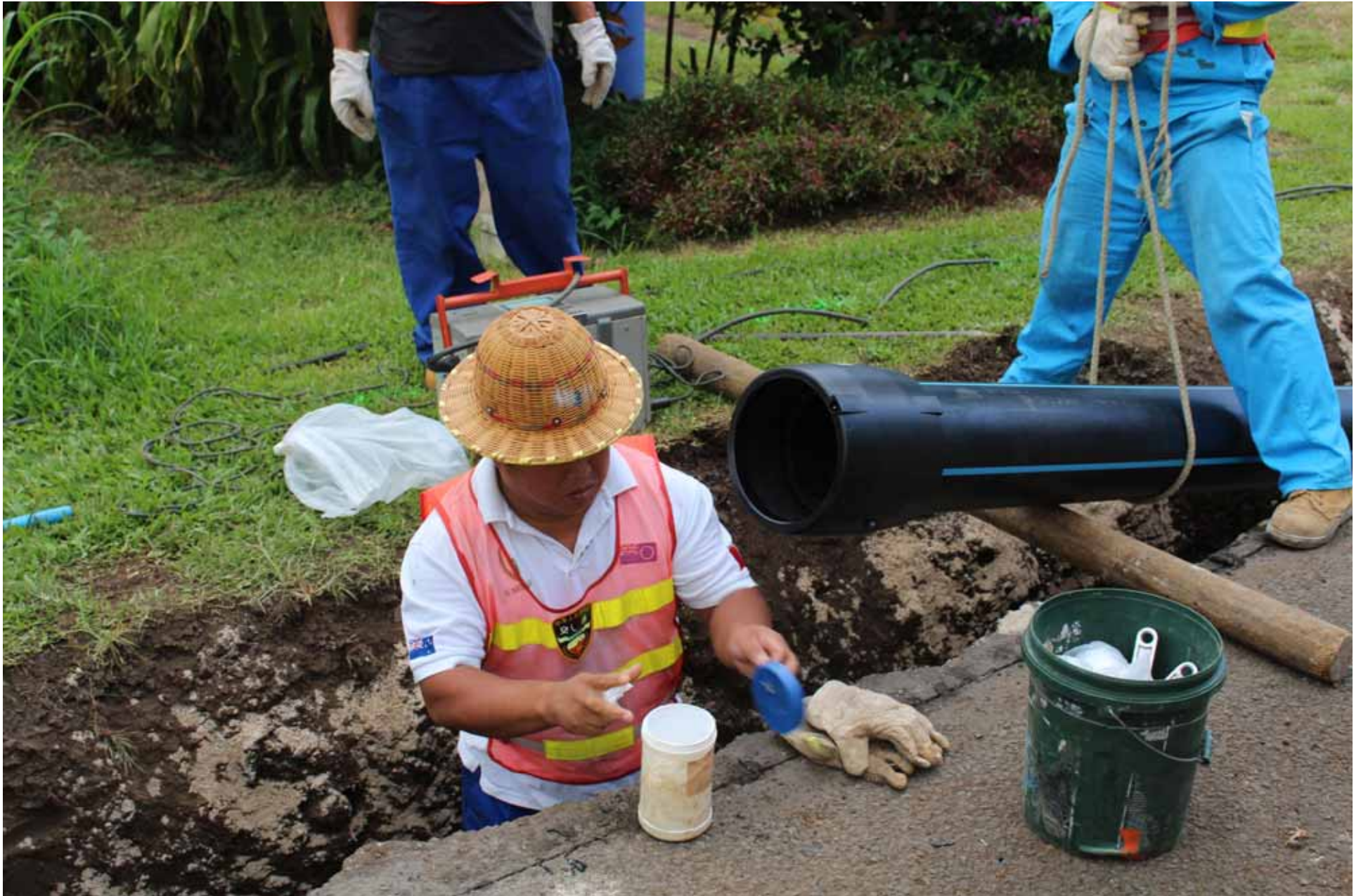
Preparing for electro-fusion welding of ring main joints by CCECC workers
