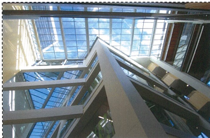
Picture 2 - Conservation House Atrium (Photo: 18/06/2009)
