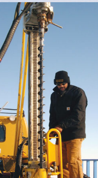
DhiresH Hansaraj drilling shot hole
