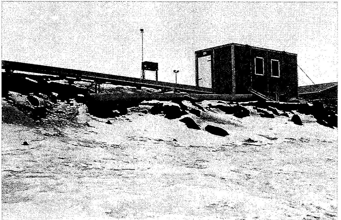
Figure 8: Wet laboratory outfall with the wet laboratory in the background, Scott Base
