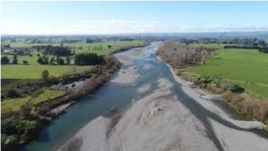
Figure 1: semi-braided channel form typical in the reach between the Rail Bridge and Fullers Bend upstream of the State Highway Bridge. Source: Waiōhine River Plan, 2020.
