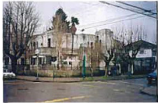
Fig. 4. Old confined masonry house currently in use in Chillán
